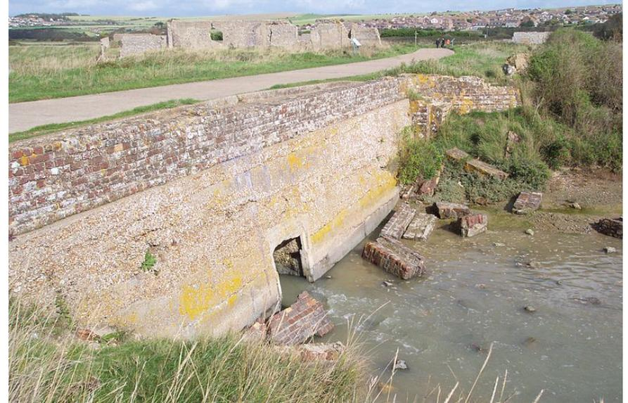
Remains of mill race sluice – left: seaward side, right: millpond side
